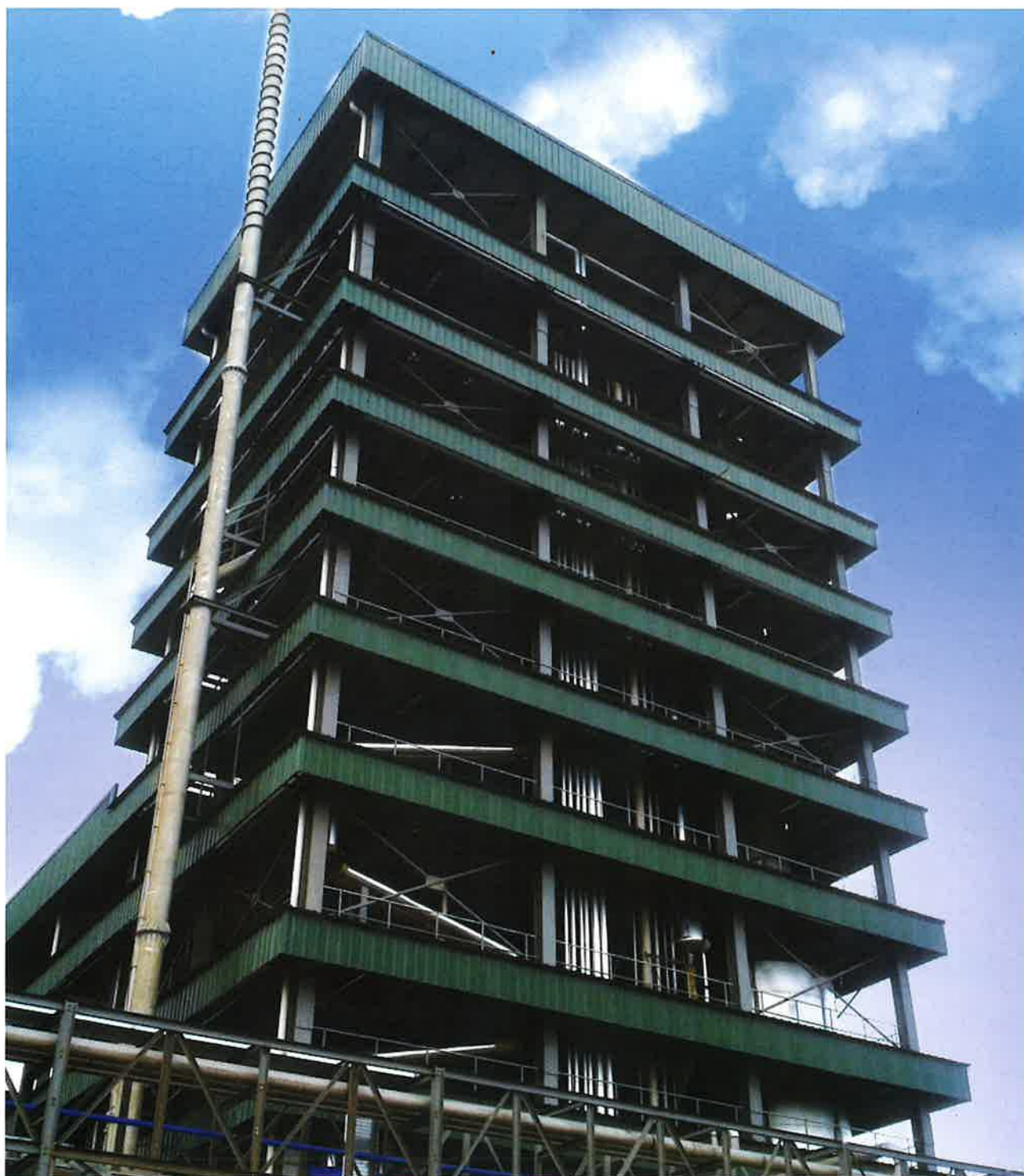
Overview of a 1,000TPD Physical Refining Plant in Sumatra, Indonesia.
